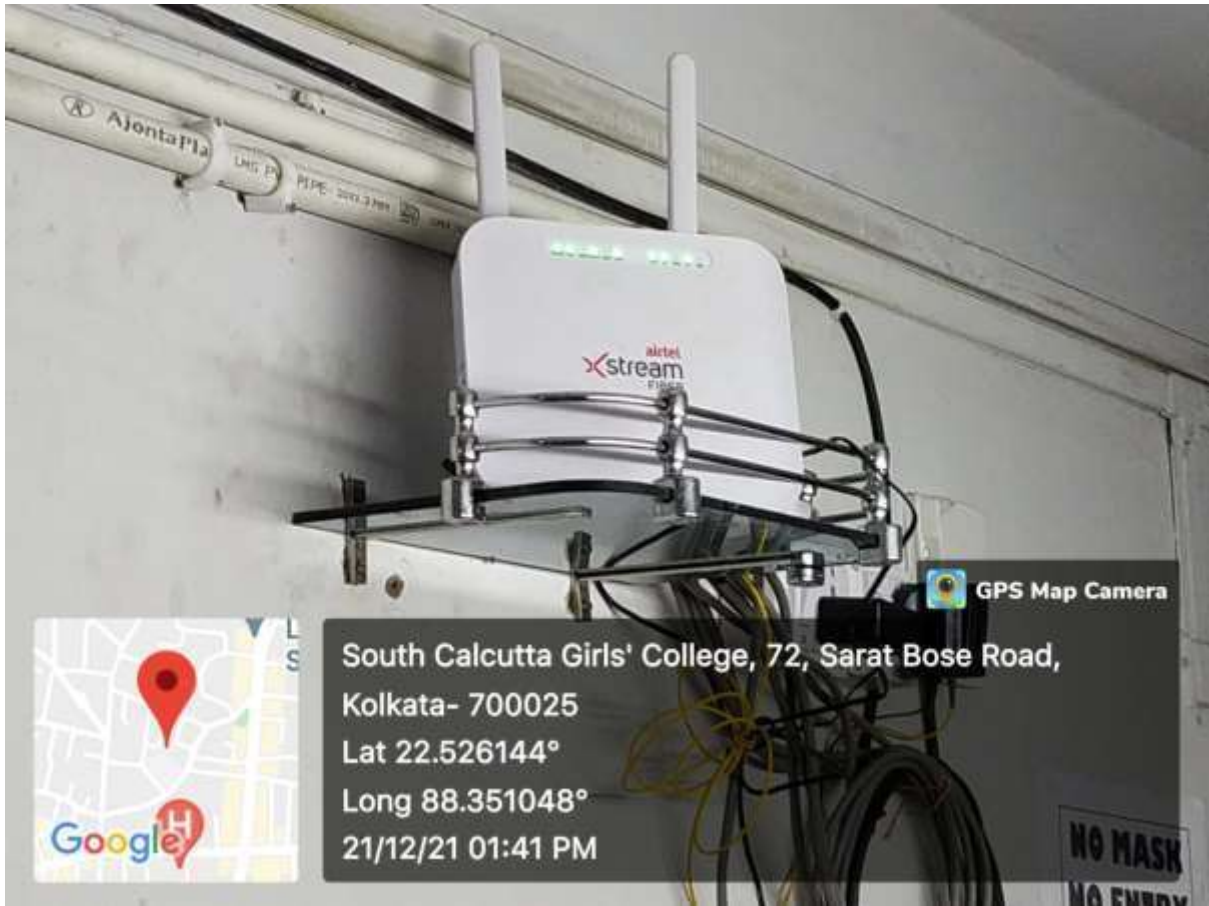
NEWLY INSTALLED Wi-Fi ROUTER FROM AIRTEL
